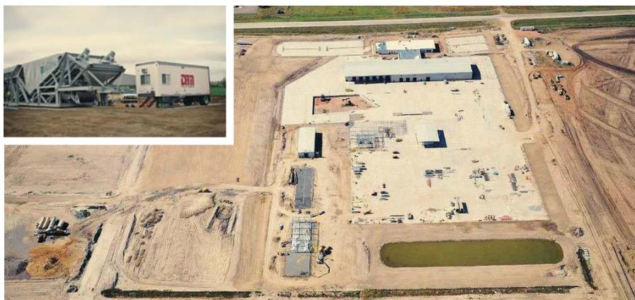
The largest project that Dickinson has poured to date is the Baker-Hughes Frac Station in 2011, which required 25,000 yd. of concrete and included seven buildings and nearly 900,000 sq. ft. of 8-in. concrete paving. This aerial shot shows the facility under construction and Dickinson's portable RexCon plant (lower-left corner) and arrival in North Dakota (inset).
